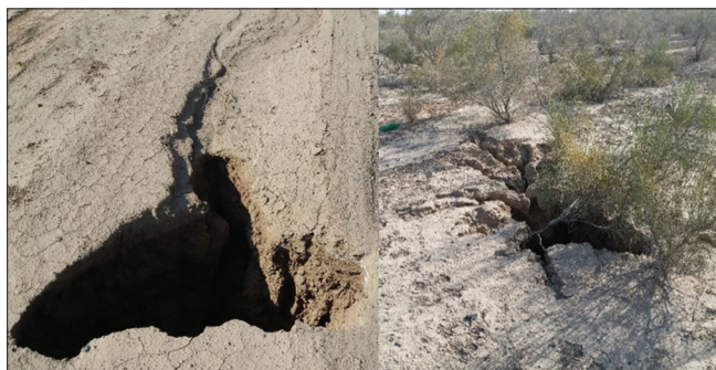
Figure 5: View of two subsidence in the study area
